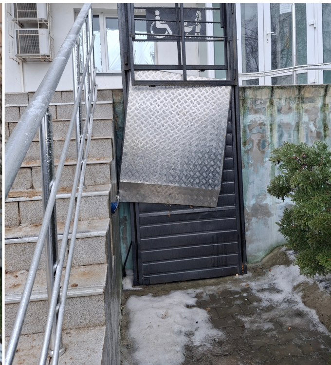
Platform lift for residents with limited mobility in a collective center in Pivdenne
