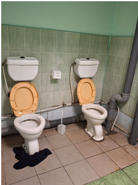
Bathroom in residential care home in Zakharivka
