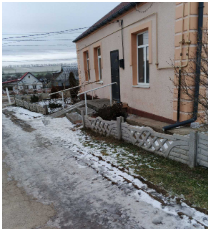
Entrance to a collective center with ramp in Stari Shompoly
