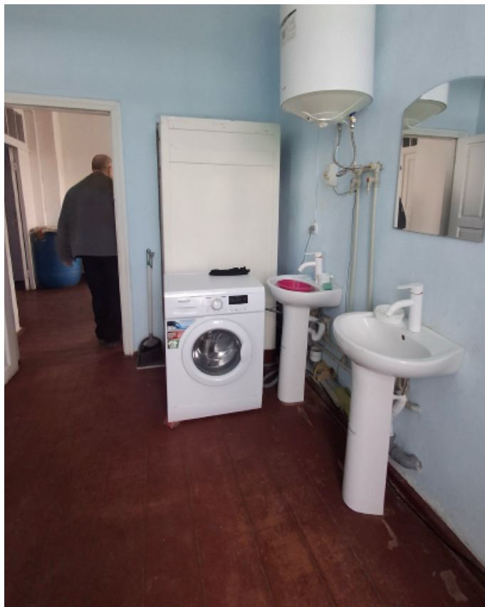
Bathroom and laundry area in a collective center in Artsyz
