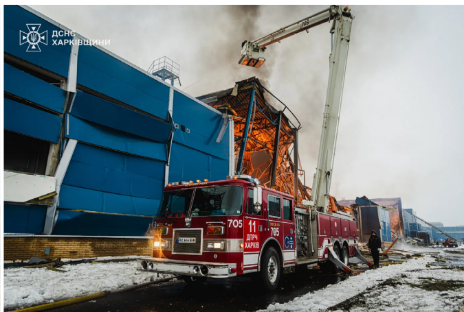
Tobacco factory warehouses destroyed by a russian missile strike Photo: State Emergency Service of Ukraine
