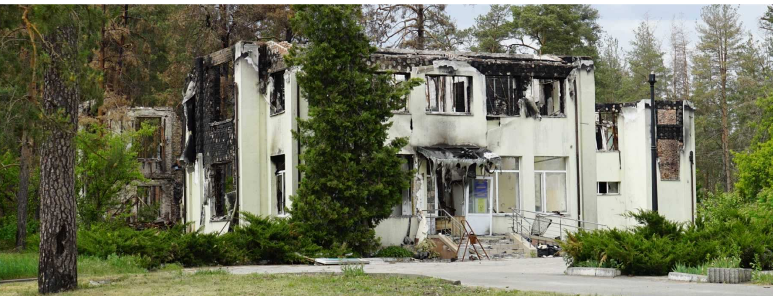
Destroyed building in Sviatohirsk, Donetsk Oblast
