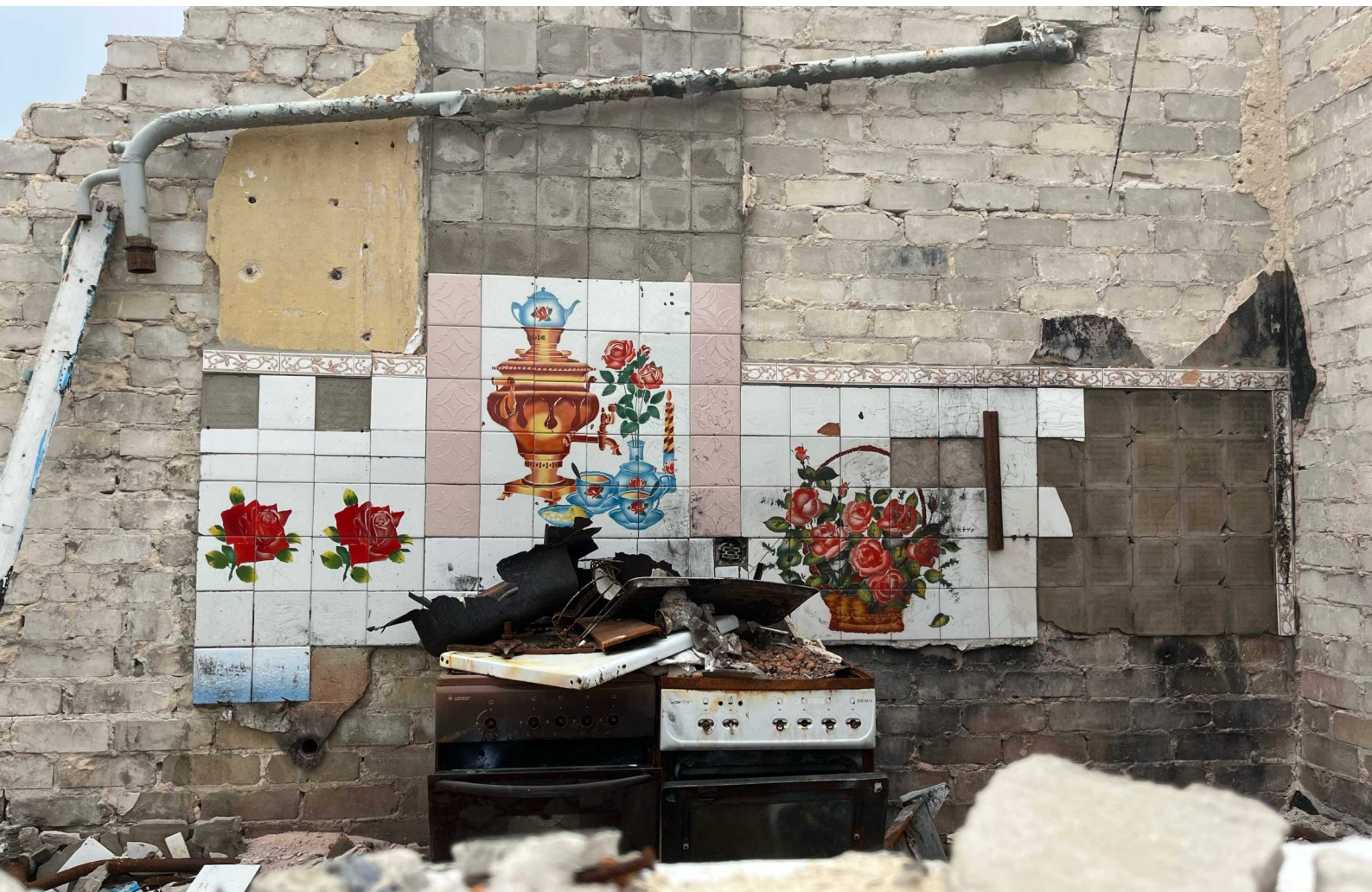
Destroyed house in Kamianka village, Kharkiv Oblast
